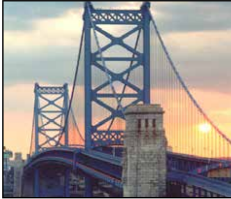
Benjamin Franklin Bridge Opened: July 1, 1926
