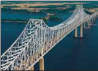
Commodore Barry Bridge
